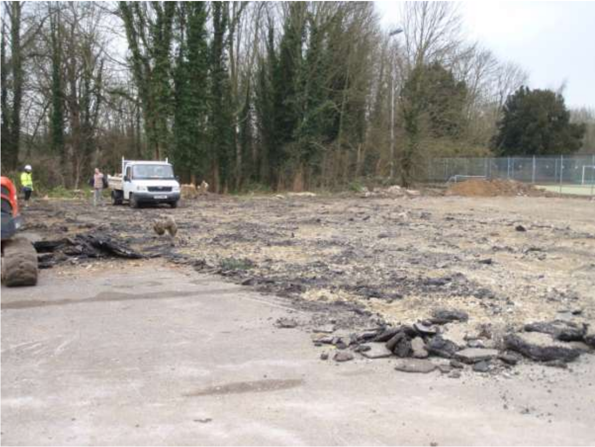
Plate 2. General view of site (Area 2) with tarmac about to be excavated, facing north
