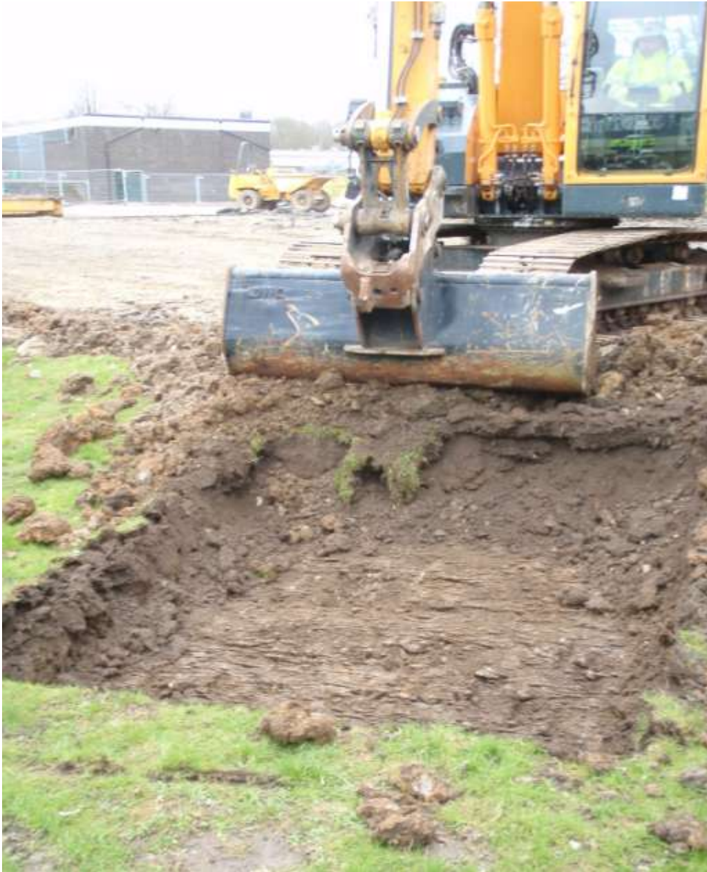
Plate 5 Excavation of soakaways (Area 2)
