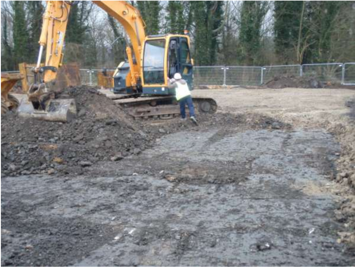
Plate 4. Area strip (Area 2) showing depth of removal required (facing south)
